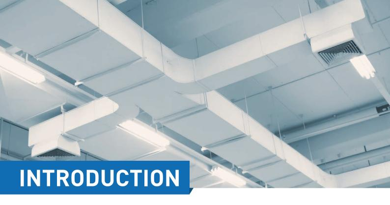
**ALPHA-PIR** air duct system is a lightweight premium quality and performance pre-insulated Polyisocyanurate air duct system for air distribution.
